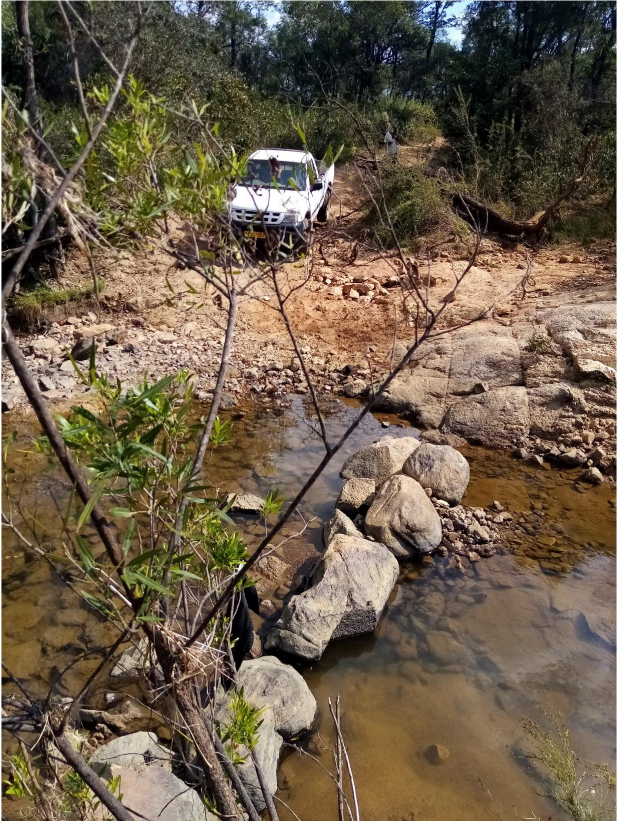
Figure 6: A typical socially produced bridge in the Innezdale community.
